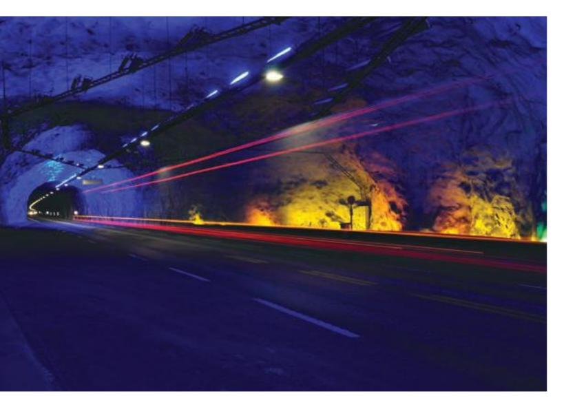
The 24.5 kilometre Laerdal tunnel is the longest road tunnel in the world. Lasting five years, work began on the tunnel in 1995, a combination of computer-controlled drilling and blasting -the latter involving the placement of a stick of Anolit dynamite in each of 100, 5 metre-deep holes for each blast- creating a 30ft diameter tube through solid rock up to 3,300ft below the surface.
